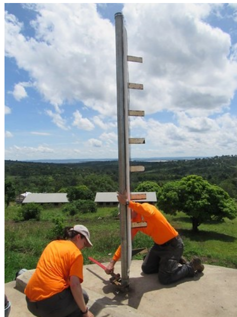
Sydney Kates (BIOE '19) and Tim McGrath (Uganda Professional Mentor) modify the Tank Level Indicator to prevent debris from entering into the tank.
