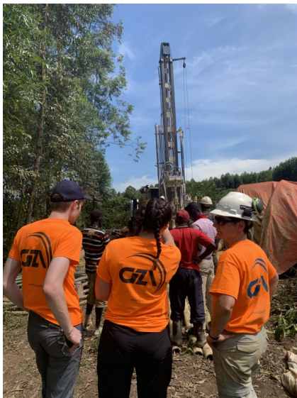
Uganda Program Members Supervising the Drilling of a Borehole from the December 2019 Implementation Trip to Nakyenyi.
