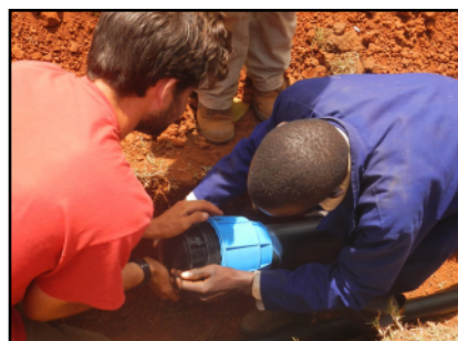
Tightening the Compression Fitting | Photo D. Saulnier
