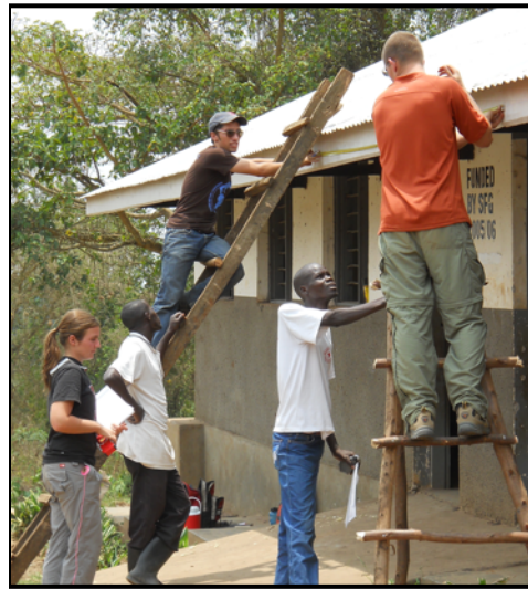
EWB members and Bbandans work on the rainwater catchment system.
