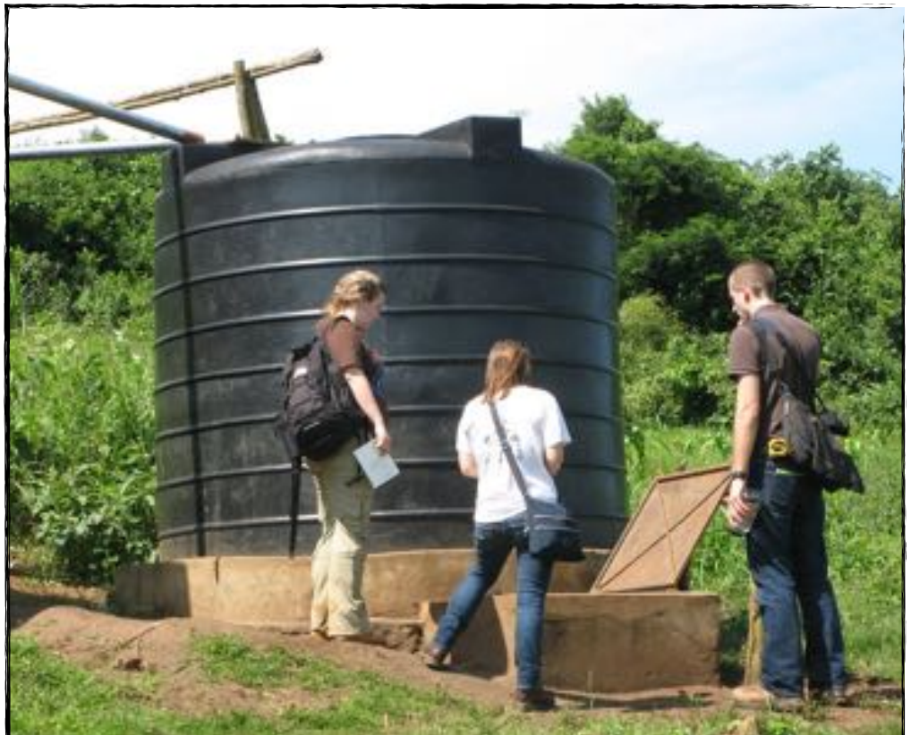
Assessing the rainwater catchment system / Photo: T. McGrath
