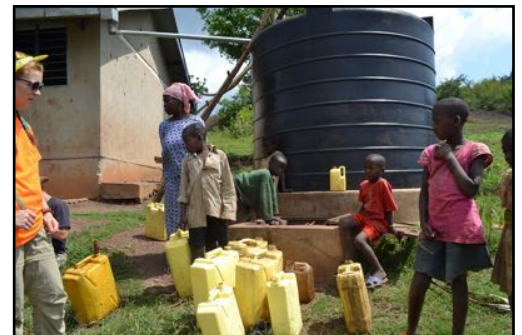
The team draining the Bbanda Umea tank so it can be cleaned, 2012 | Photo: L. Cherchia
